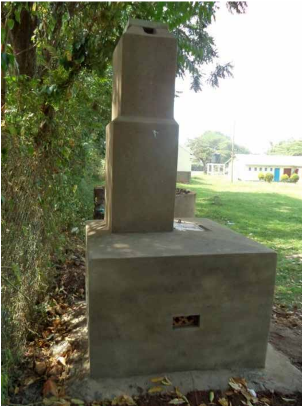
In 2015 we constructed an incinerator at the RHU Mbale clinic
